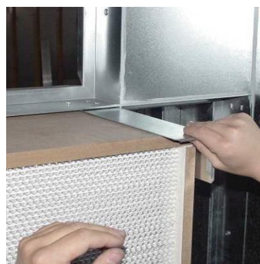
Figur 158: Sett inn filtercellen
