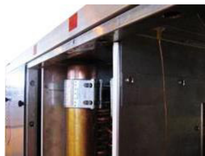
Figur 175: Montert STRAUB-kobling
