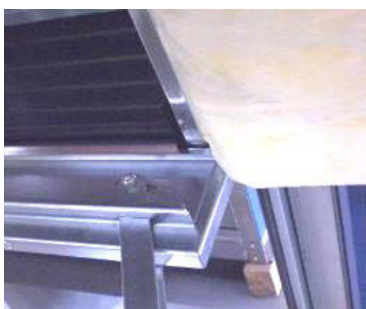
Figure 145: Slide in the filters
