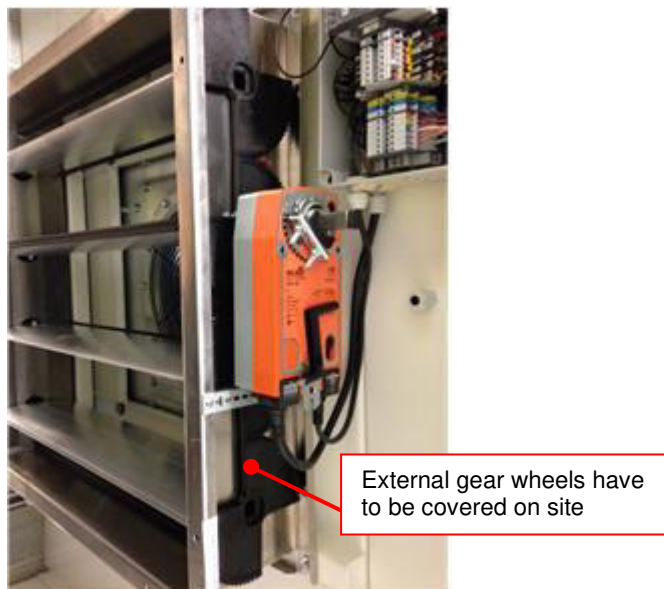
Figure 163: Damper with external gear wheels
