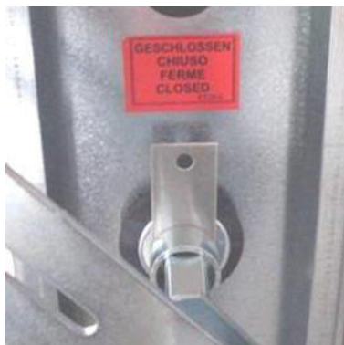
Figure 137: Closed position, characterized by a sheet metal position indicator
