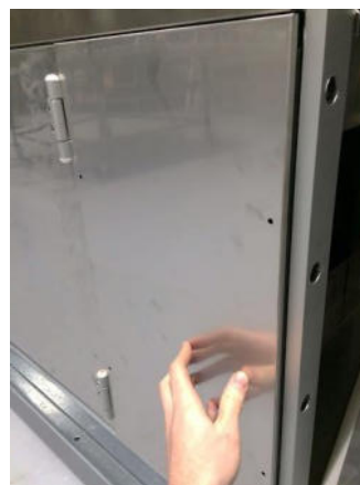
Figure 90: Outer panel not screwed
