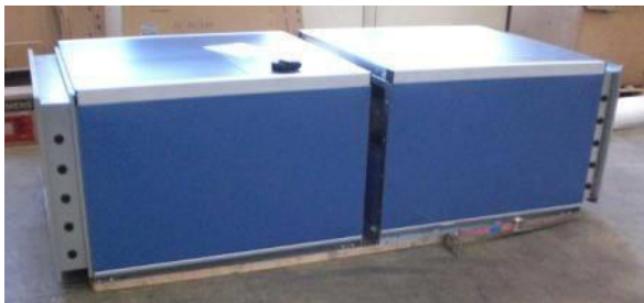
Figure 49: Pulling AHU sections together
