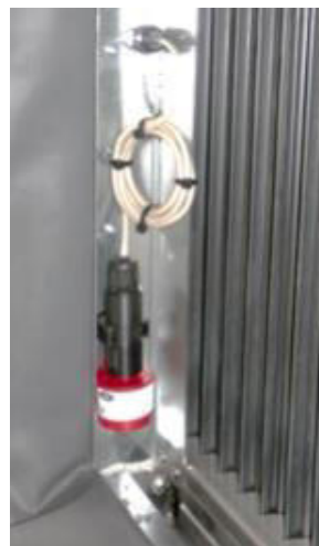
Figure 166: Mounted gas detector
