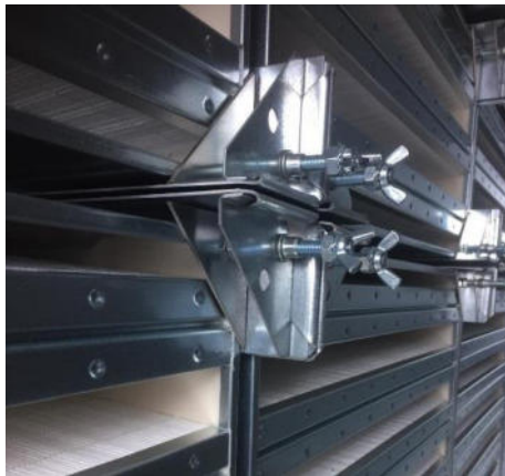
Figure 157: Filter tensioner with pressure plate
