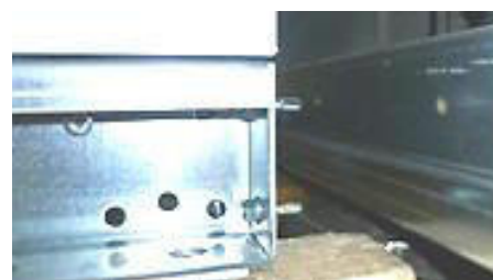
Figure 73: Application of self-tapping screws
