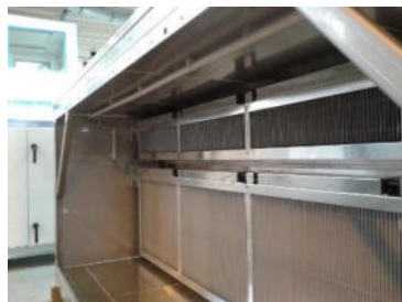
Figure 161: Electrostatic filters in the filter frame
