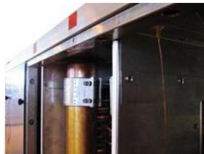
Figure 171: Mounted STRAUB coupling
