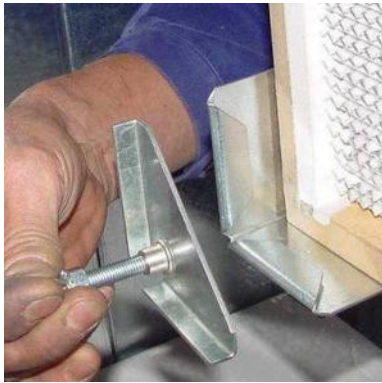
Figure 155: Inserting the clamps
