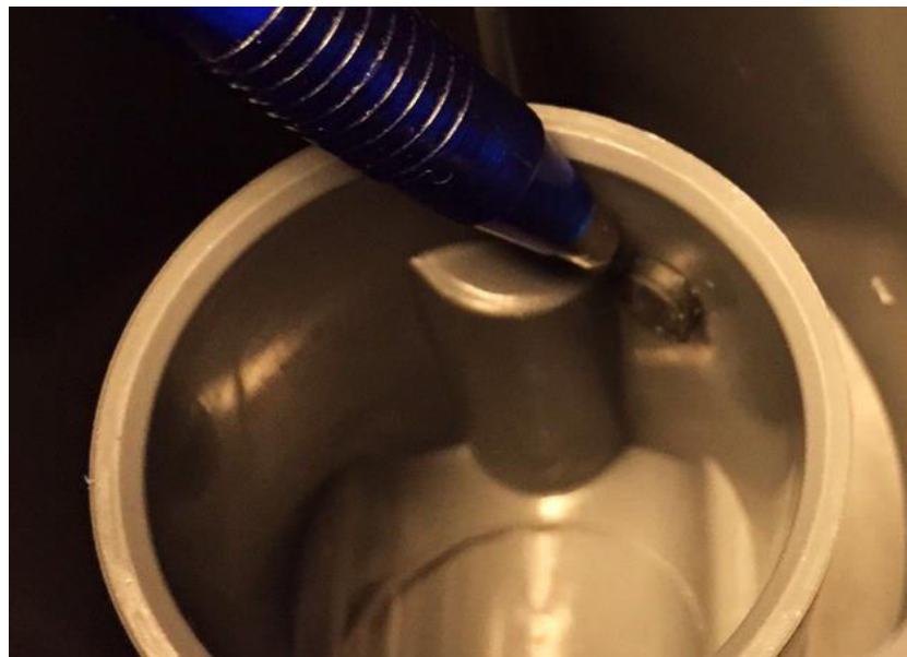
Figure 188: Pressure side installation: remove the black closing plug
