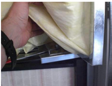
Figure 147: Lifting the filter bags
