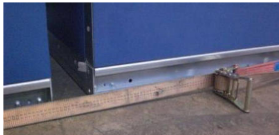
Figure 50: Pulling AHU sections together (detail)
