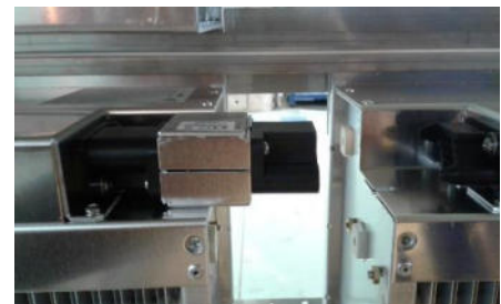
Figure 162: Plug connection electrostatic filters
