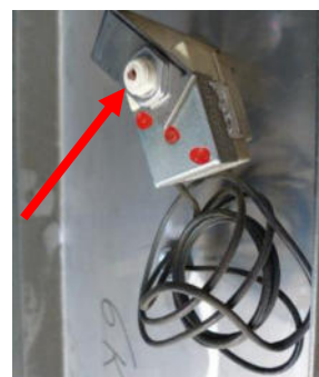
Figure 202: Thermostat with uncovered reset button
