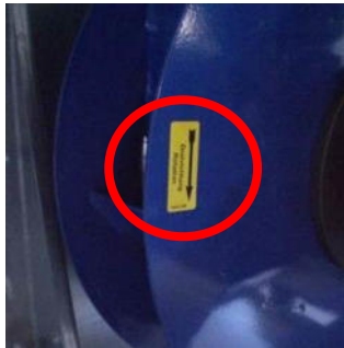
Figure 196: Rotation marking of plug fans
