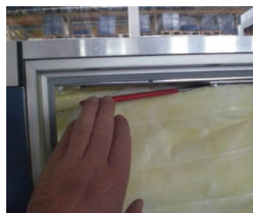
Figure 146: Clamping the filters
