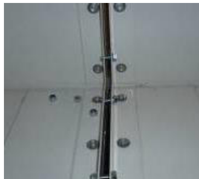
Figure 64: Connection via connection strengthening angle
