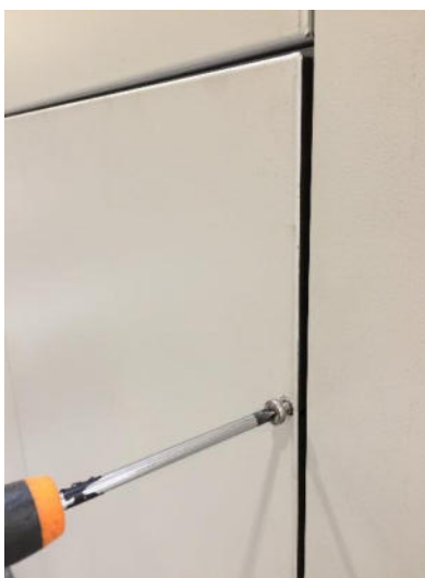
Figure 130: Undoing the screw and removing the door panel (TRA-E) from the door frame
