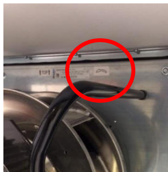
Figure 198: Rotation marking of EC fans
