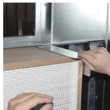
Figure 154: Inserting the filter cell
