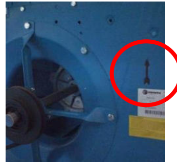
Figure 197: Rotation marking of housing fans
