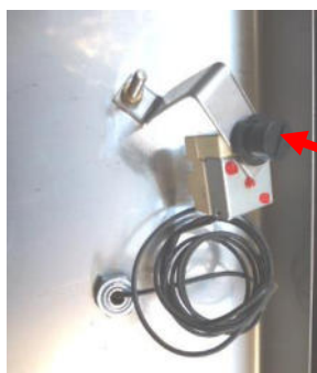
Figure 201: Thermostat with cover cap on the reset button
