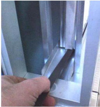
Figure 139: Pulling out the filters
