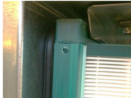
Figure 152: Check, if filter lie on the sealing
