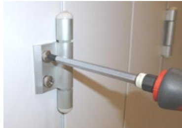
Figure 121: Adjustment of the door panel (EU.T)
