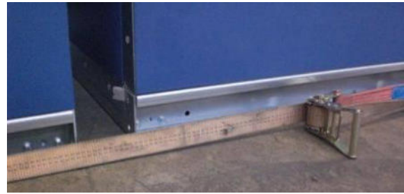
Figure 23: Pulling AHU sections together (detail)
