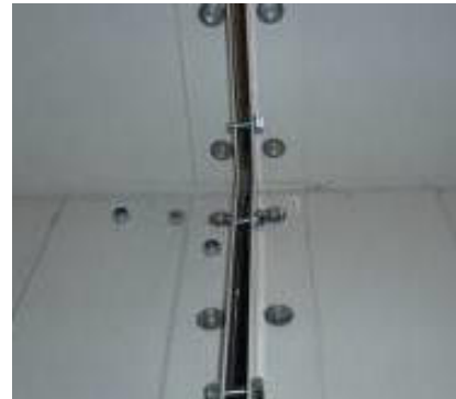
Figure 30: Connection via connection strengthening angle
