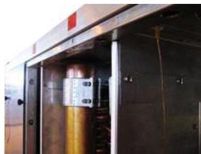
Figure 60: Mounted STRAUB coupling
