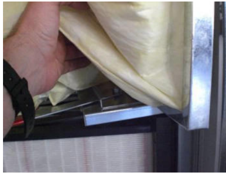
Figure 47: Lifting the filter bags
