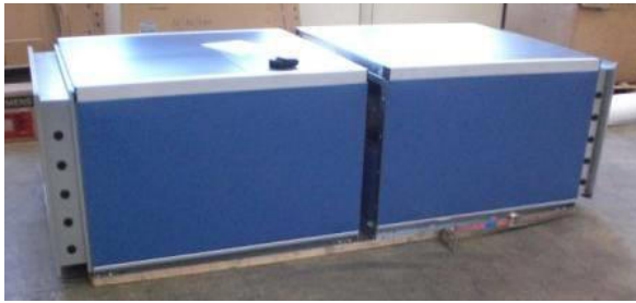
Figure 22: Pulling AHU sections together
