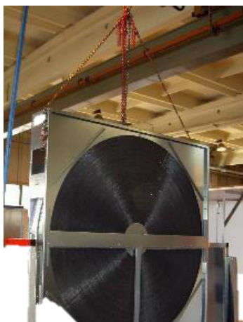
Figure 83: Lifting with chain hoist
