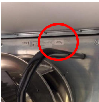
Figure 72: Rotation marking of EC fans
