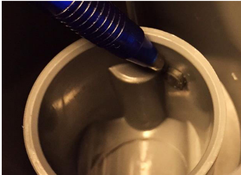
Figure 70: Pressure side installation: remove the black closing plug
