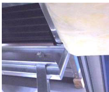
Figure 45: Slide in the filters
