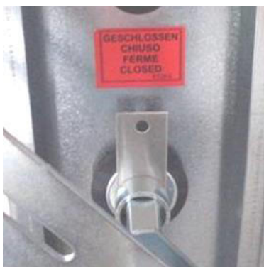
Figure 42: Closed position, characterized by a sheet metal position indicator
