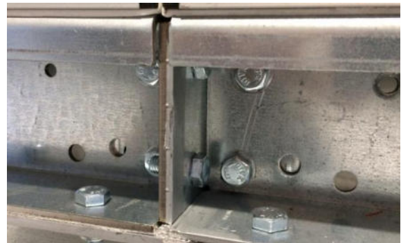
Figure 25: Bolt connection of base frames
