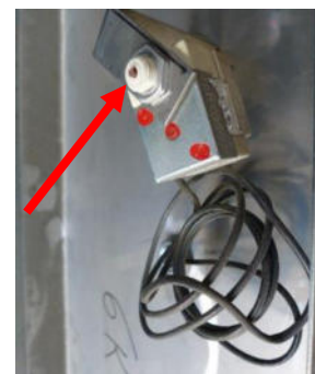
Figure 75: Thermostat with uncovered reset button
