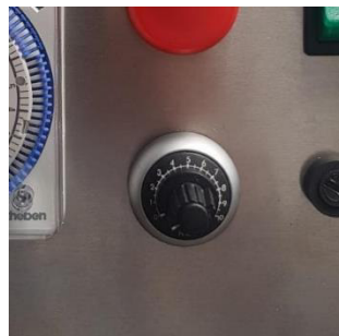
Figure 12: Mounted Potentiometer on the side of the AHU
