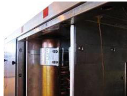
Illustration 172 : raccord STRAUB monté
