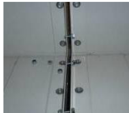
Illustration 64 : Raccordement via un angle de raccordement
