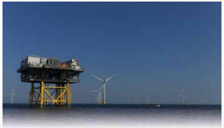
Off-shore platforms WORLDWIDE
